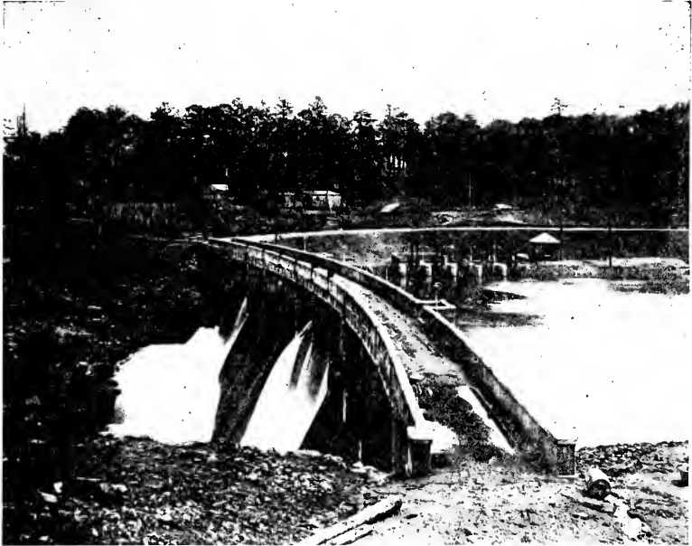
FIG. 52.—Tunnel Intake, Showing Its Relation to the Diversion Dam.
